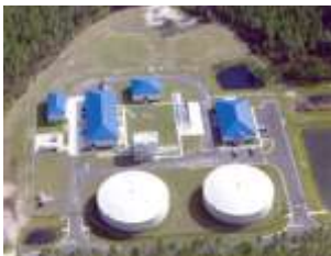
Price Creek Water Plant
